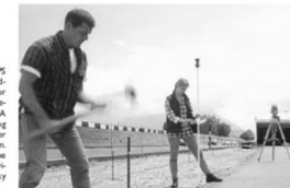
FIGURE 5.26 Leica TPS System 1000, used for road-way stakeout. The surveyor is controlling the remote-controlled total station (TCA 1100) at the prism pole using the RCS 1000 controller together with a radio modem. The assistant is placing the steel bar marker at the previous set-out point. (Courtesy of Leica Geosystems Inc.)
